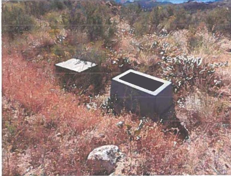
**Photograph 1. Electrical conduit was run to the building sites under the previous owner. However, electrical service was never installed.**
